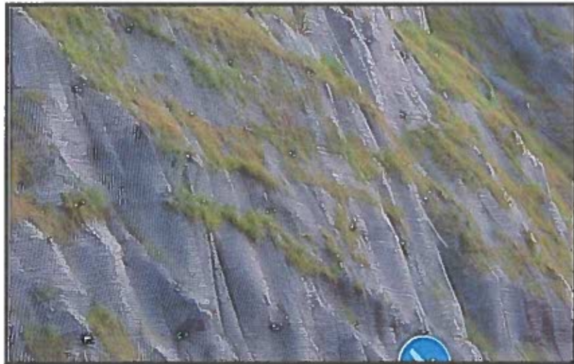
Photograph 1 – Example of Geobrugg TECCO slope stabilization system in place
