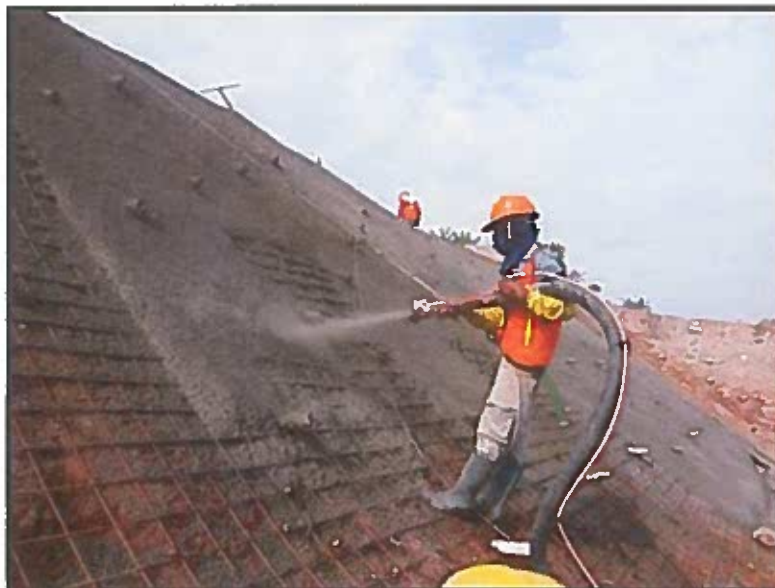
Photograph 2 – Example of Concrete Face Hillside Stabilization
